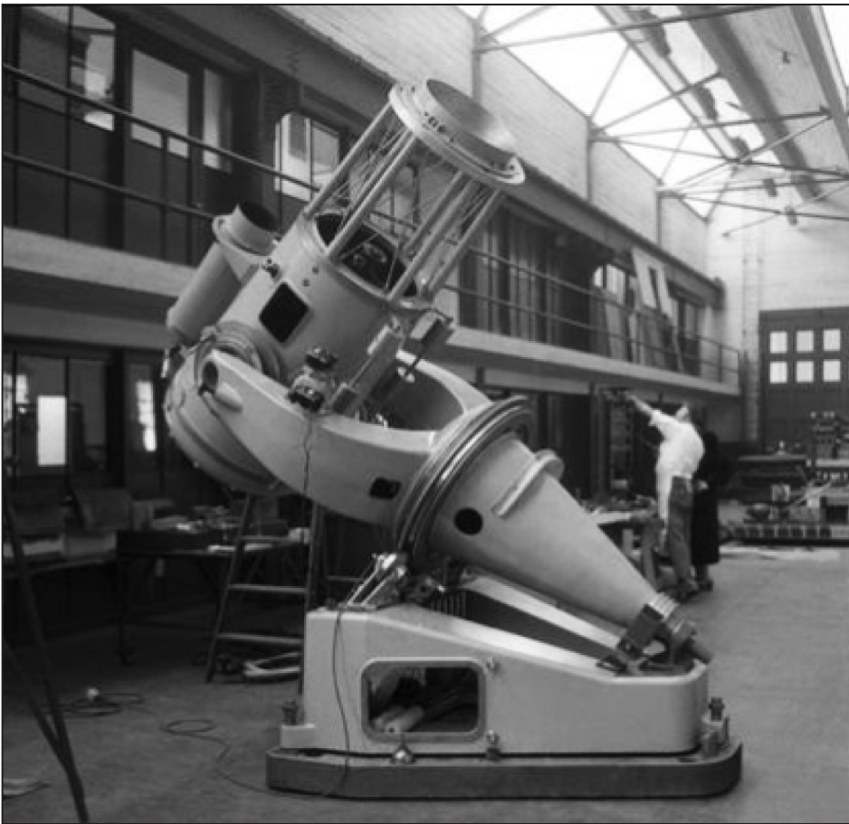
The 18-inch Schmidt as photographed by F. Ellerman during its fabrication in the Caltech Instrument Shop, 1936 (Palomar/Caltech/Caltech Archives)
